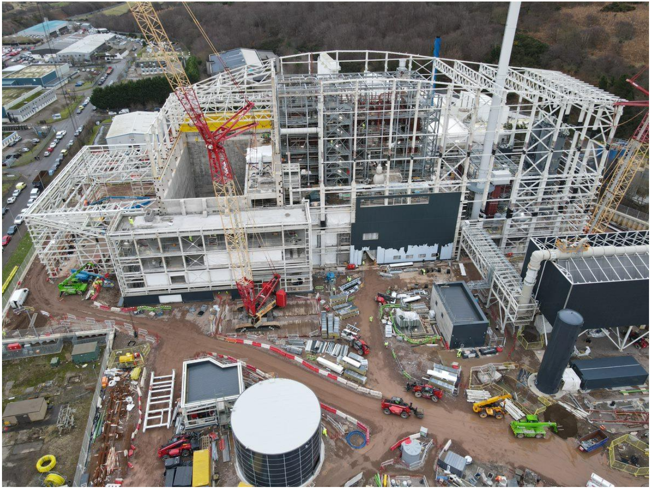
View from West of Facility: Note Bunker complete and Cladding commencing
