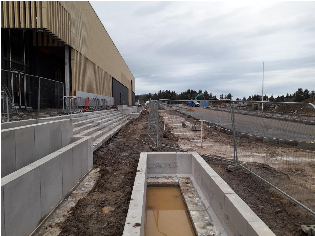
Photograph 1 Main approach to front of building – photograph taken w/c 29 th November 2021
