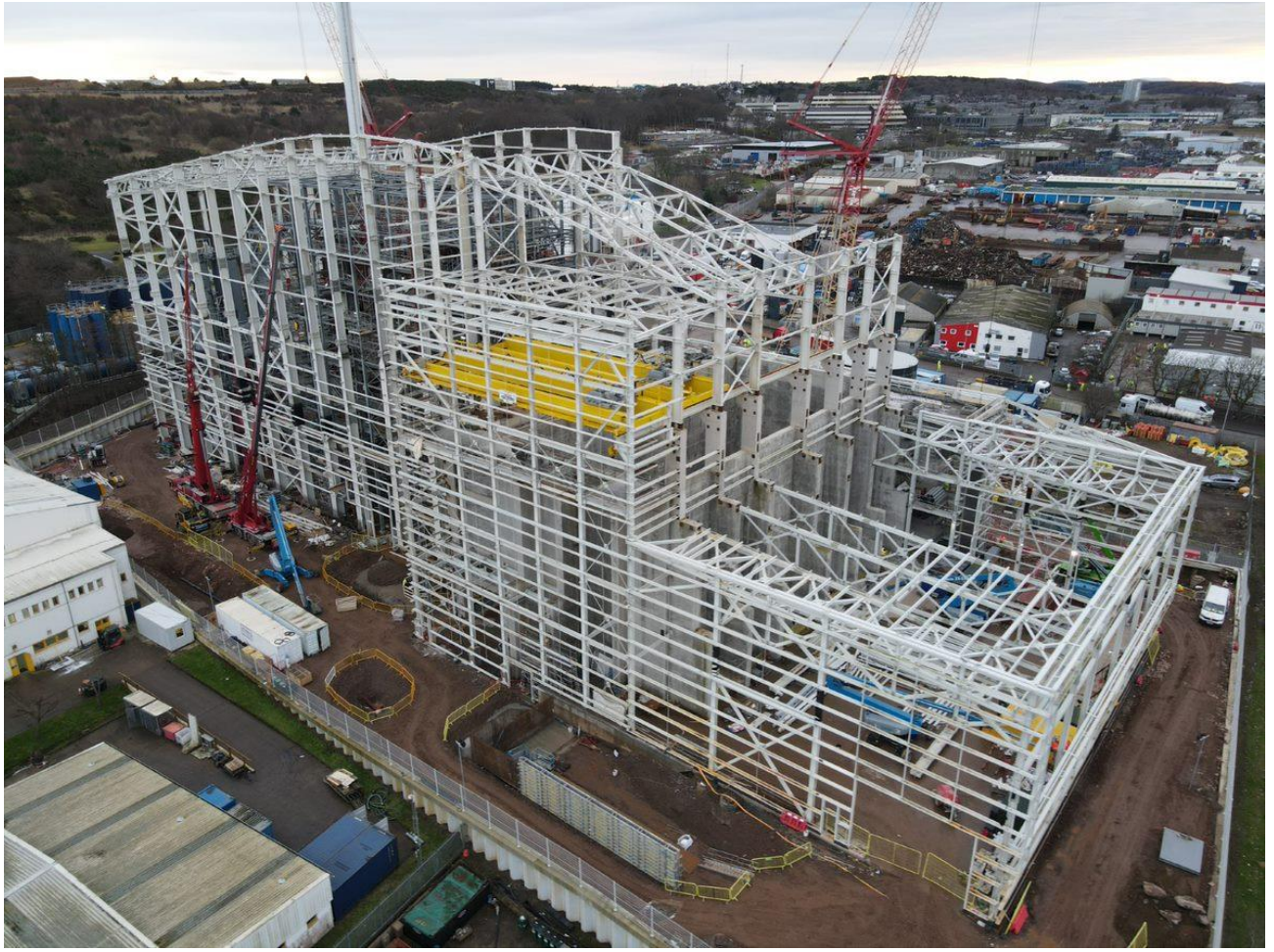
View from Northeast: Main Building Steelwork shape becoming apparent
